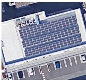
Tenryu Factory #2 40 kW (from 2018)
