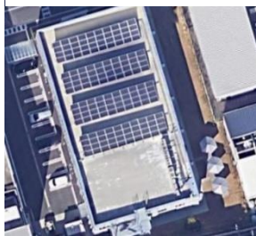
Tenryu Factory #1 90 kW (from 2017)
